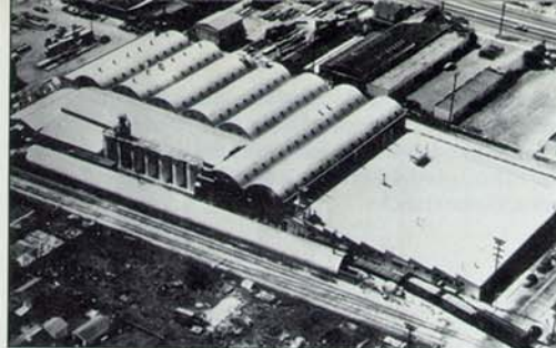
RIGHT: Aerial view of the Tepco factory built in 1947 after a fire destroyed the original plant. Note the clay-filled train pulling up to the Tepco spur. BELOW: The batter-out (right) and the jiggerman at Tepco, ca. 1947. Each team "threw" about 200 dozen pieces a day.
